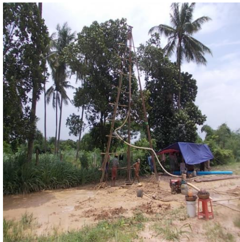
Figure (9). Photograph shows manual water jetting with mud circulation drilling method
